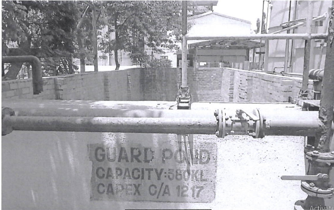
Guard pond of 380 KL capacity
